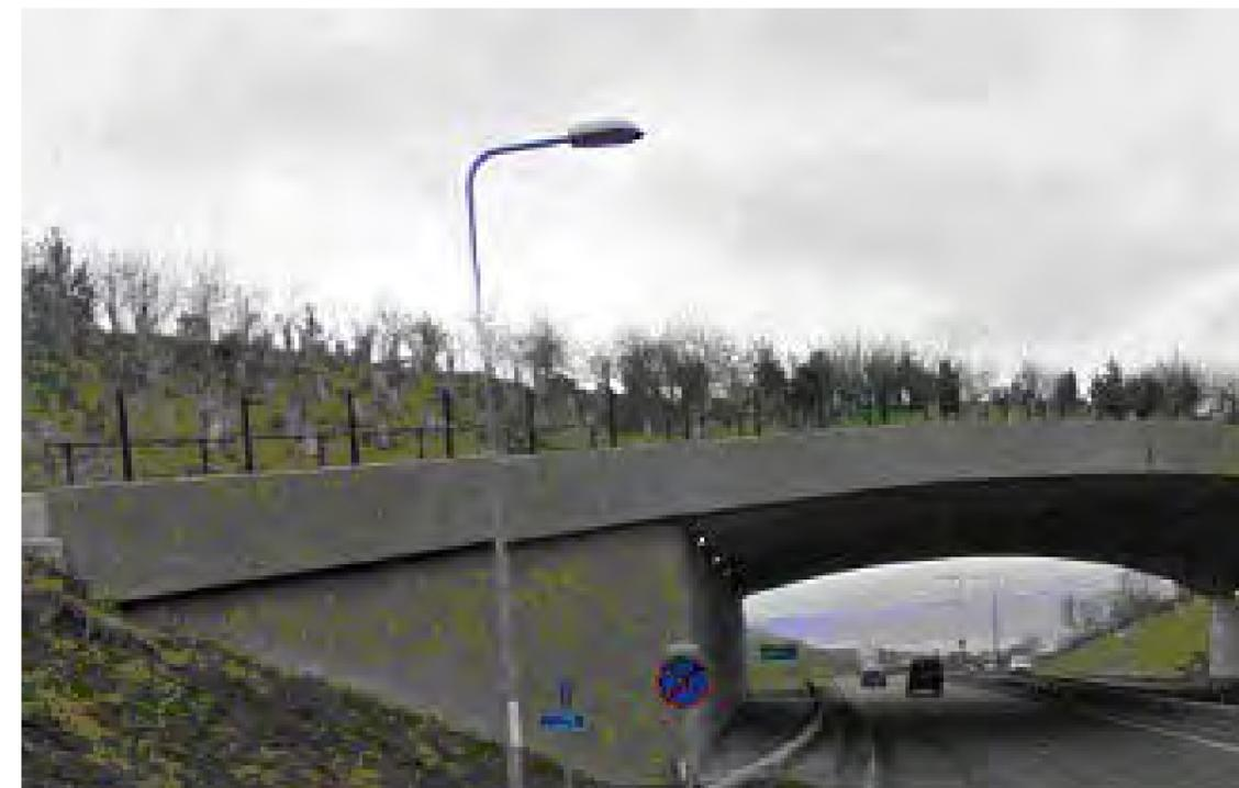
Figure 237: The green bridge over the A21 near Scotney Castle in Kent is seamlessly integrated with the context and allows for wildlife to cross.
